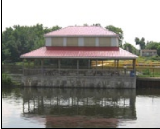
A photo of the gazebo located on Lock Island.
