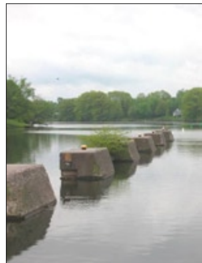
The installation of floating docks alongside these concrete impoundments is one recommendation of the VRC.
